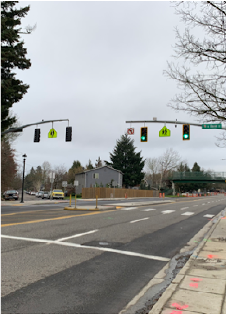
Pedestrian crossing light with the HAWK signal.
